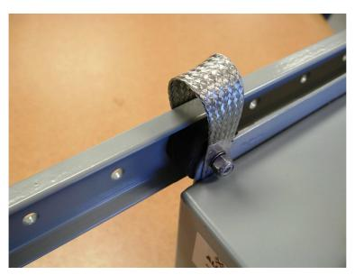
Once the strap is installed correctly, the assembly should look like the photo to the left.
